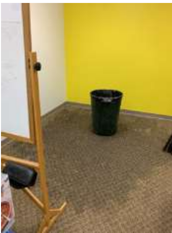
Water damage in a classroom from an ice dam
